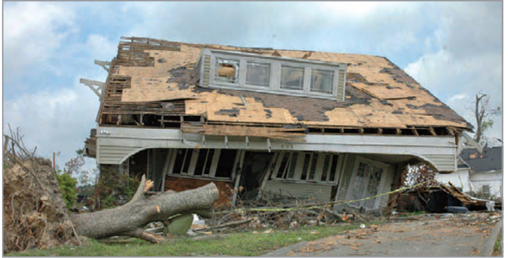
Marshall House (Ca. 1905), 601 4th St., Cullman Historic District
